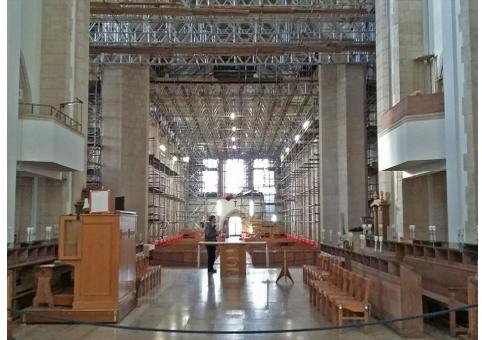
weight is being suspended from the walls – an engineering feat! This is necessary to protect both the underfloor heating system and the floor itself, which were put in after the vault had been completed. The scaffolders are to be congratulated for rising to a very real challenge. It is worth a visit!
